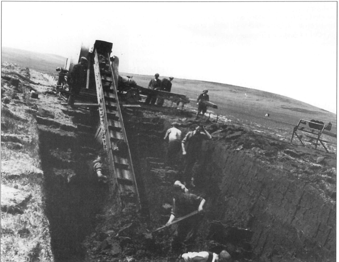
Figure 3.20: Loading an Akermann peat macerating machine. Eleven of these machines were bought by Bord na Móna in the late 1940s under Todd Andrews, but only a few were used.
